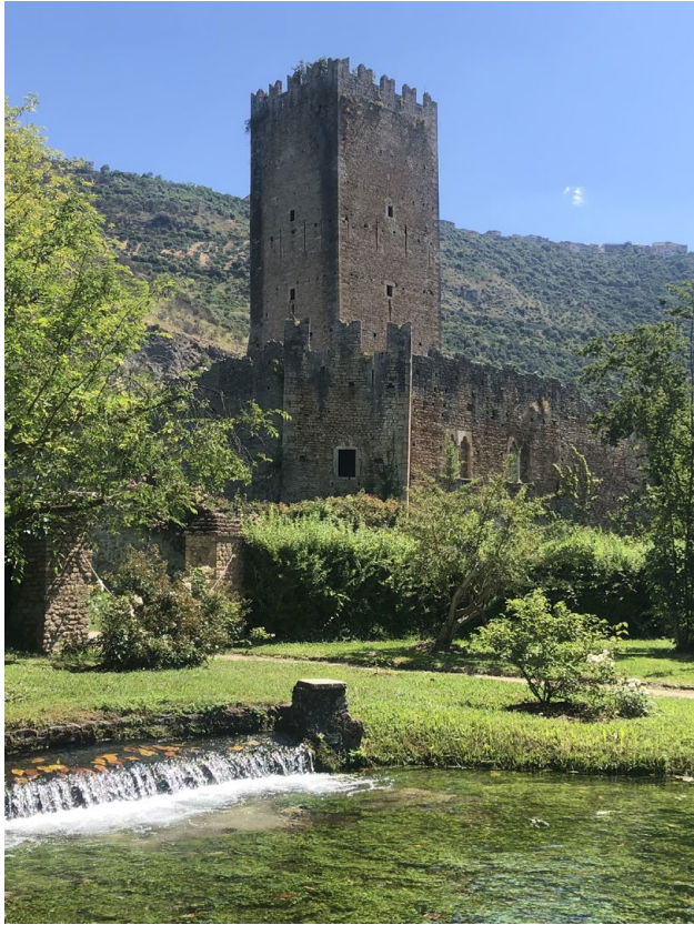
Fig. 7. Remains of the Medieval city of Ninfa – a typical wall designed and set as if it were a kind of opus caementicium (picture: Roberta Fonti).
