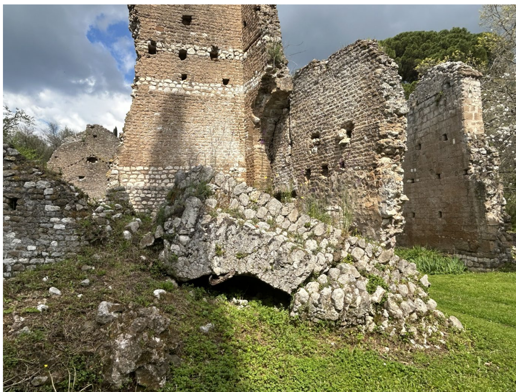
Fig. 8. Remains of the Medieval city of Ninfa – an historical collapse of a wall out-of-plane (picture: Roberta Fonti).
