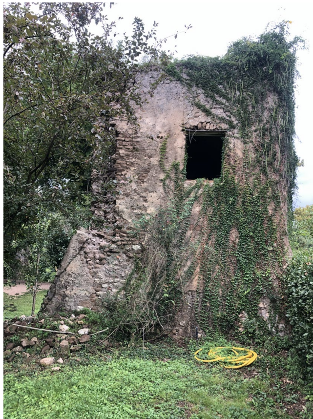
Fig. 10. Remains of the Medieval city of Ninfa – (a) historic picture showing the roof of this tower house freshly painted with a white lime-wash (picture: with the courtesy of the Fondazione Roffredo Caetani); (b) the same tower house (year, 2022) showing an out-of-plane mechanism of collapse of its quoin and possessing an arched construction in its indoor space; and (c) a tree reaching its life cycle (pictures: Roberta Fonti).
