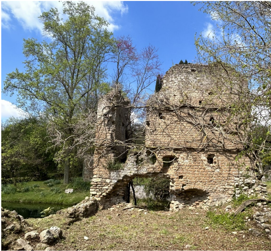
Fig. 9. Remains of the Medieval city of Ninfa – a wall held out-of-plane by the help of the vegetation (picture: Roberta Fonti).
